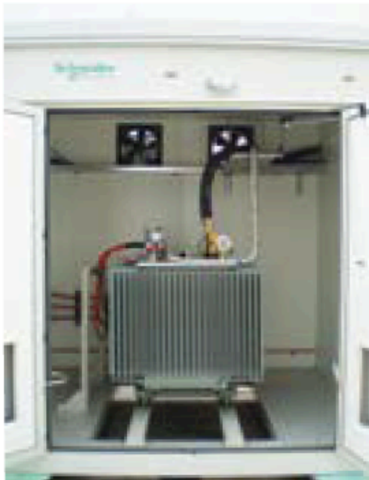
Transformer in PV box
