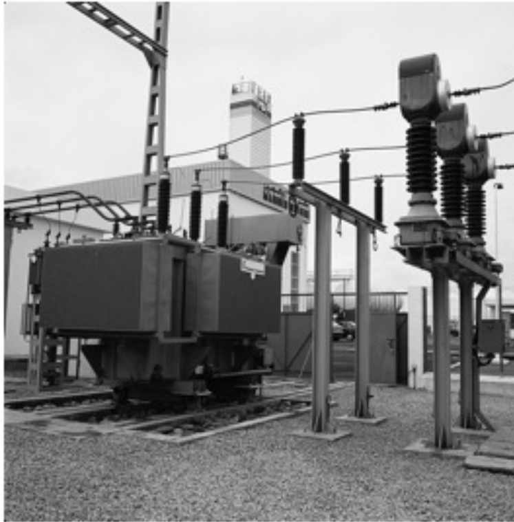
Air-breathing conservator-type tank at atmospheric pressure
